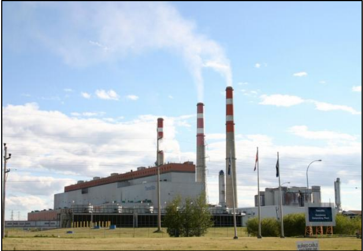
FIGURE 4: SUNDANCE COAL FIRED GENERATION STATION (WEIS, THIBAUT, PARTINGTON, GIBSON, & ANDERSON, 2012)
