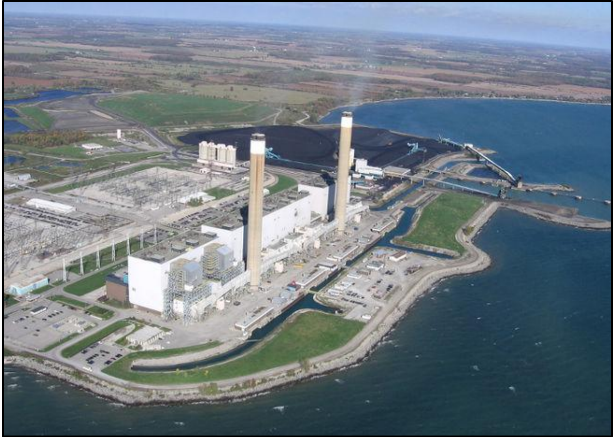
FIGURE 3: NANTICOKE POWER GENERATING FACILITY IN NANTICOKE ONTARIO. ONCE THE LARGEST COAL FIRED PLANT IN NORTH AMERICA AT 4 GW PEAK CAPACITY, HAS BEEN DECOMMISSIONED AS OF DECEMBER 2013 (WEIS, THIBAUT, PARTINGTON, GIBSON, & ANDERSON, 2012).
